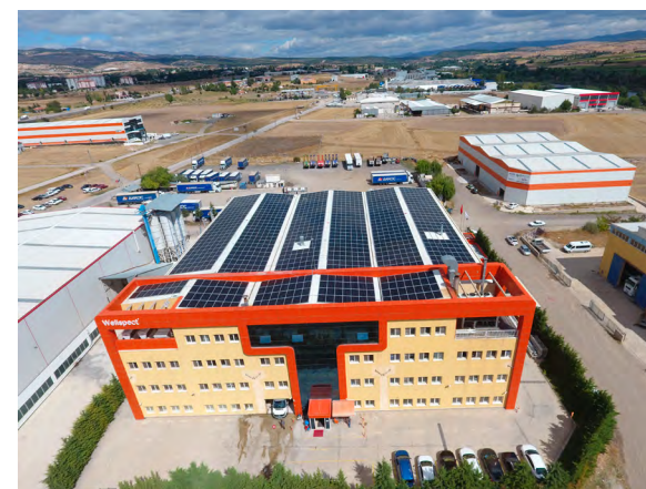
Renewable energy installations at our manufacturing sites, such as our facility in Kazan, Turkey, help support our efforts to reduce GHG emissions
